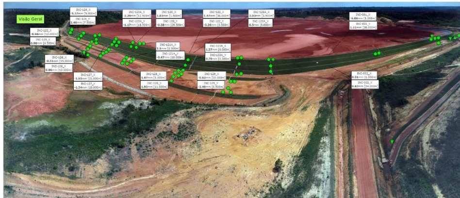
Figure 7. B1 dam geotechnical monitoring.
