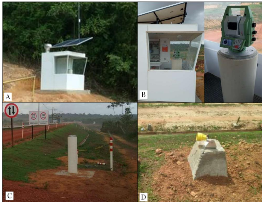
Figure 5. a) Cabins topographic monitoring, b) Robotic Monitoring Total Station (RMTS), c) Reference mark and d) Monitoring prism.
