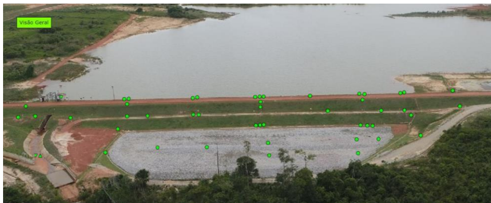
Figure 9. B6 dam geotechnical monitoring.
